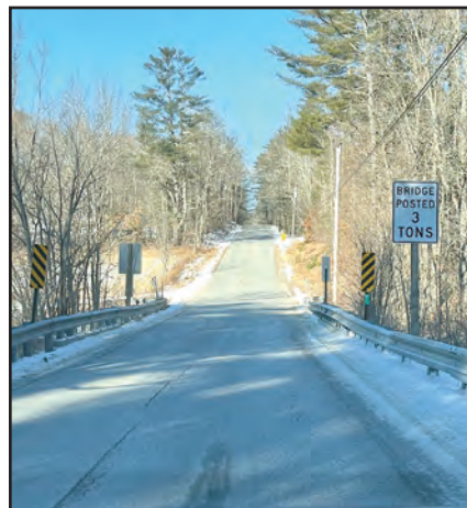
Varney's Bridge on William Knight Road over the Pleasant River in Windham will be replaced by MDOT this summer at a cost of $2.07 million as part of their Three Year Plan. PHOTO BY ED PIERCE
