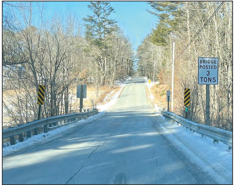
There will be a detour for about a month on Varney's Bridge on William Knight Road in Windham this summer as bridge replacement work will be performed. Motorists are advised to use Falmouth Road or Route 302 to get around the bridge construction. PHOTO BY ED PIERCE
