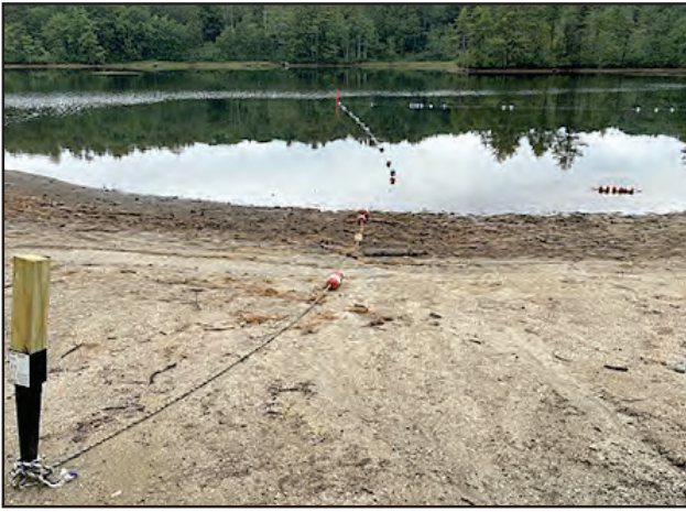
A malfunction of the Dundee Hydroelectric Dam gate has caused a swimming ban at Dundee Park until further notice. COURTESY PHOTO
